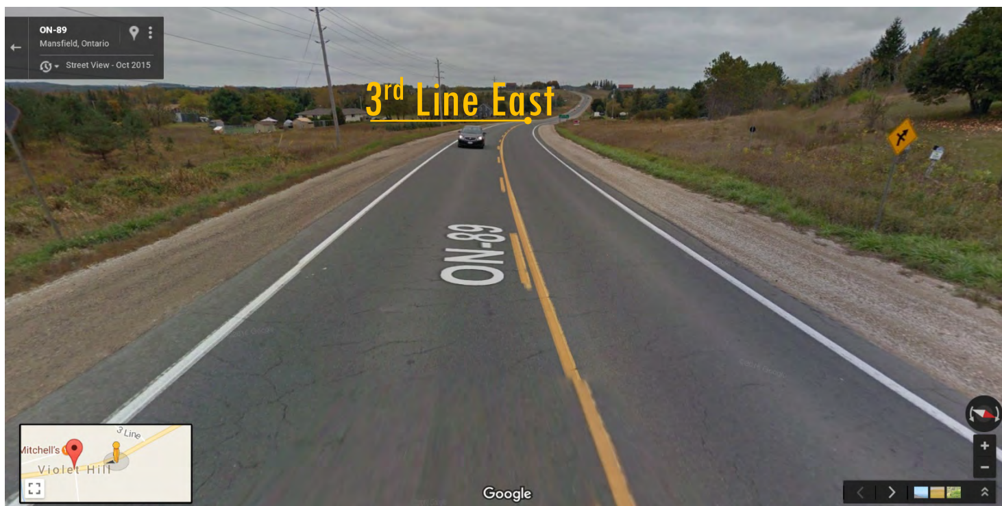
looking west to 3 rd Line East from 185 metres to the east
