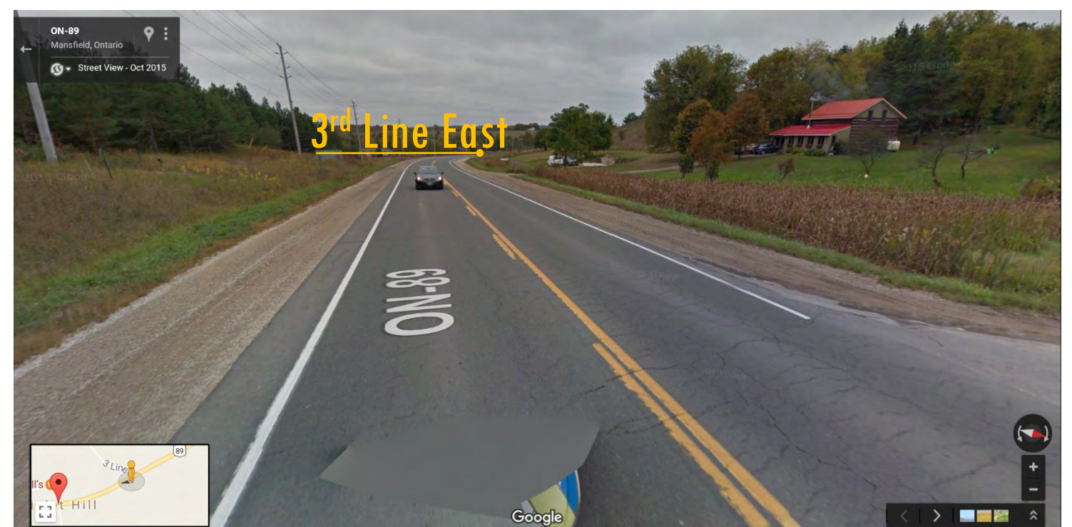
looking west to 3 rd Line East from 320 metres to the east
